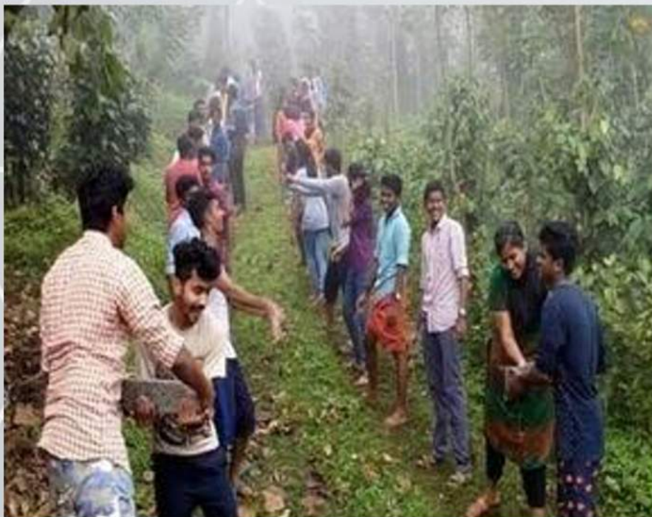
Road Construction at Kannampady(15/09/2016)
