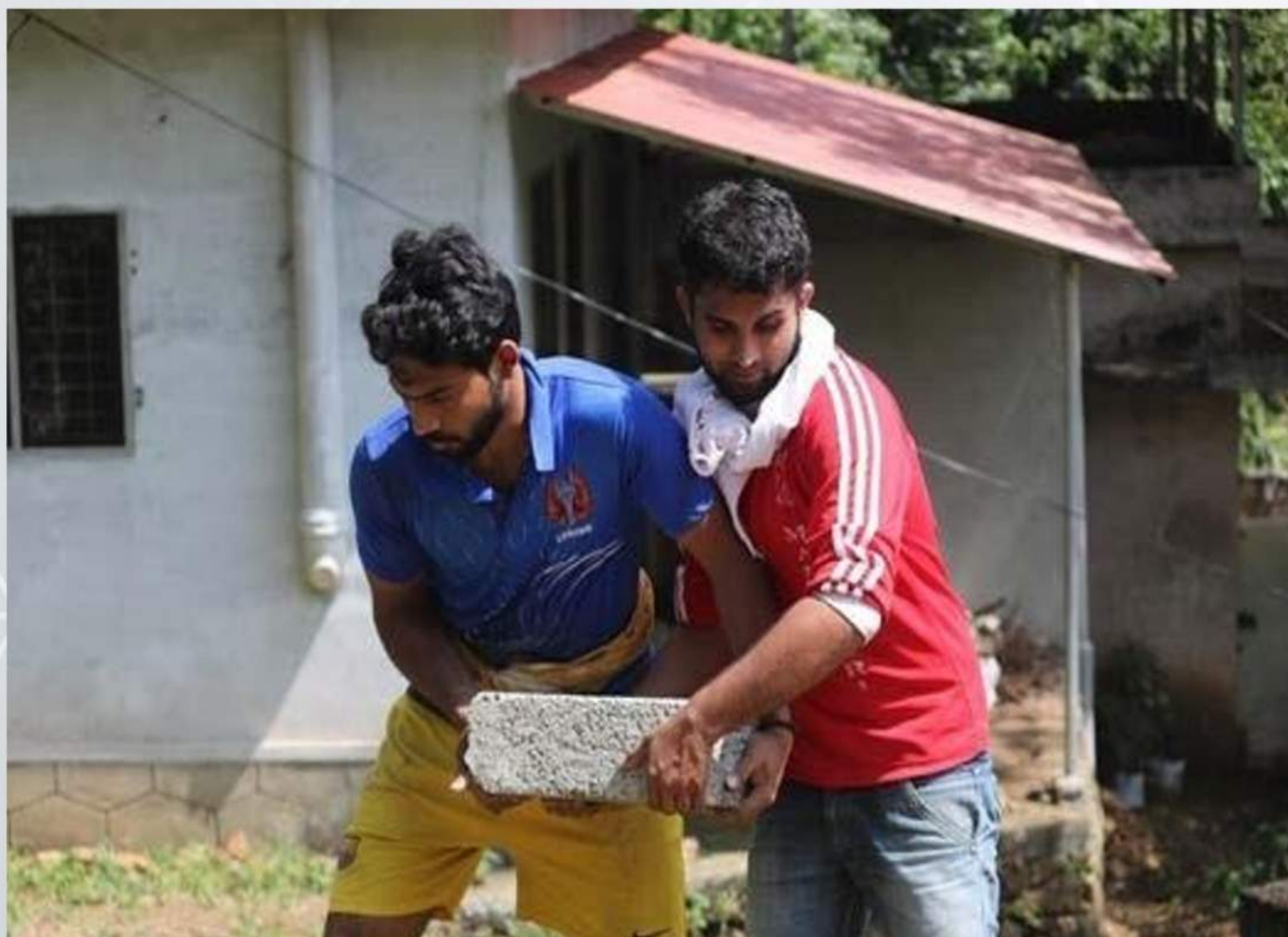
Cleaning Premises and House Construction (21/09/2016)
